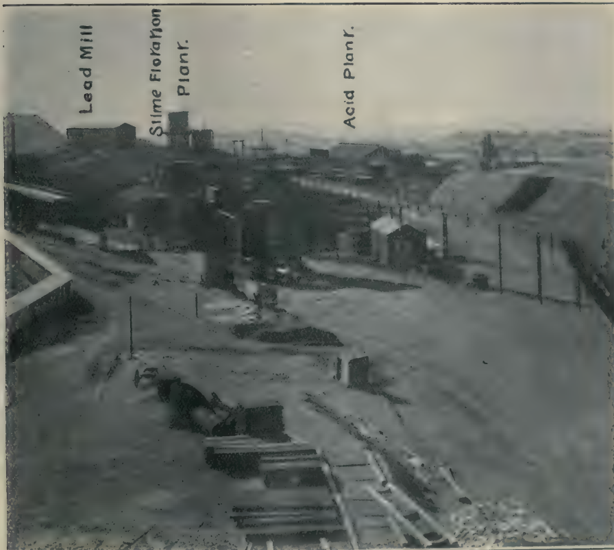
SOUTH MINE, LOOKING NORTH-EAST.
